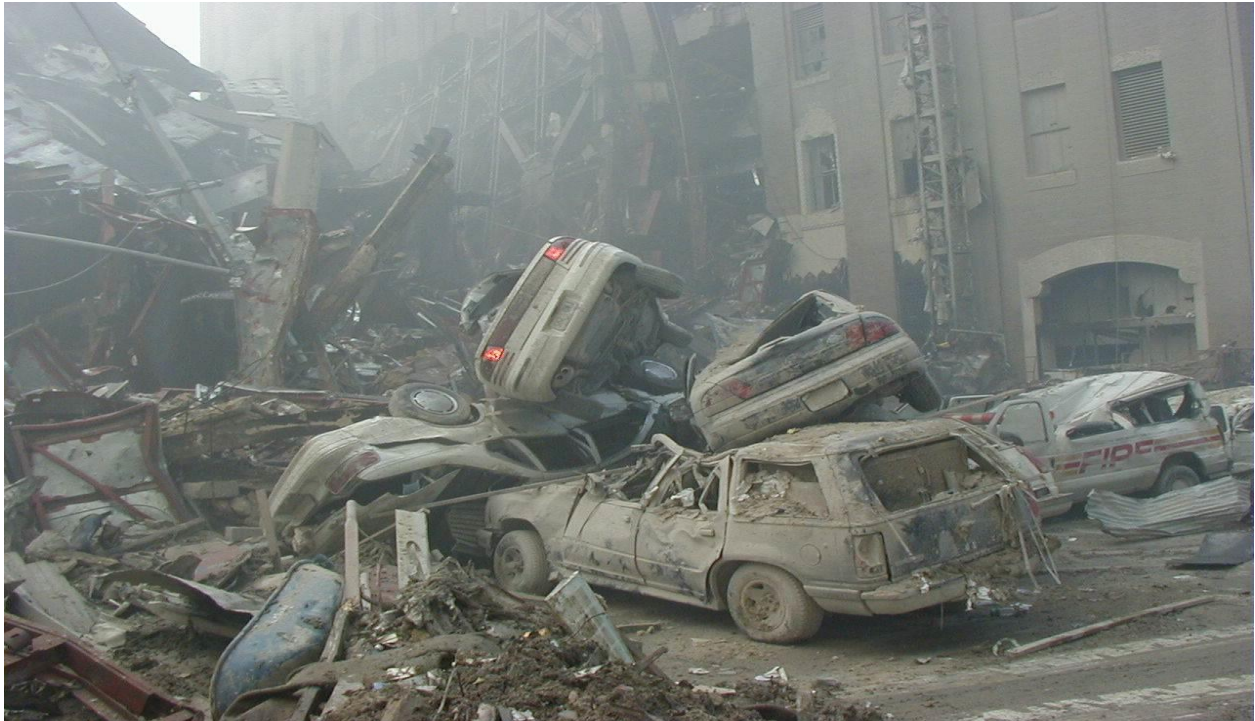
Dirty bombing of Federal Building; fire, MCI, building collapse; hazmat release
