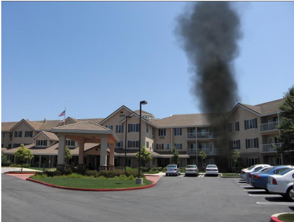
Fire in assisted living facility due to disgruntled employee – unknown whereabouts
