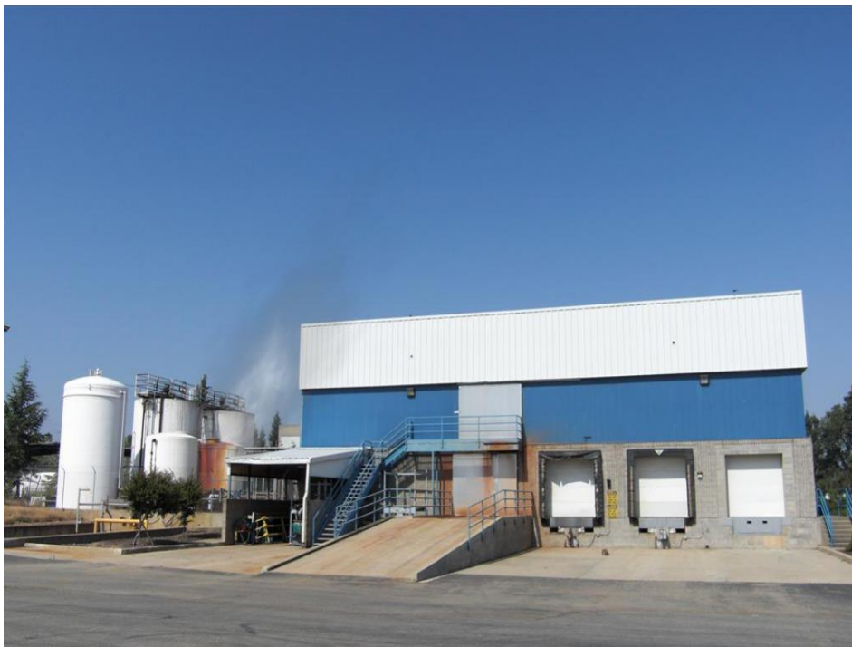
Hazardous material leak in an industrial complex
